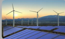
Wind Power Inverters
