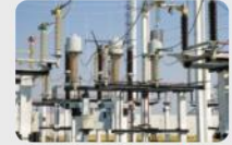
Sensor & communications gateway
